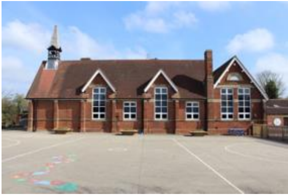
Woolpit Primary School (Bell Tower)
